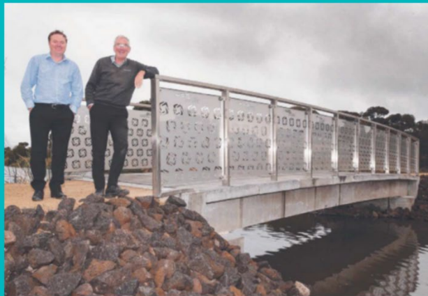
Kevin Foard and Austeng's Ross George inspect the city's non-corroding bridge
